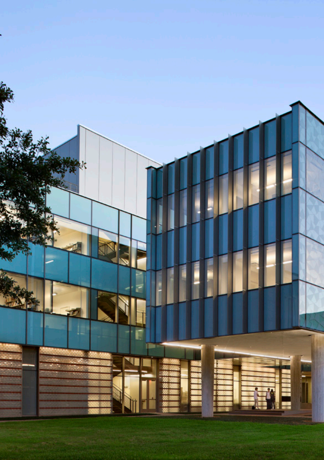
Fig 2.3 Glass and aluminium curtainwall at Brockman Hall for Physics at Rice University, Houston, Texas, USA, designed by KieranTimberlake
