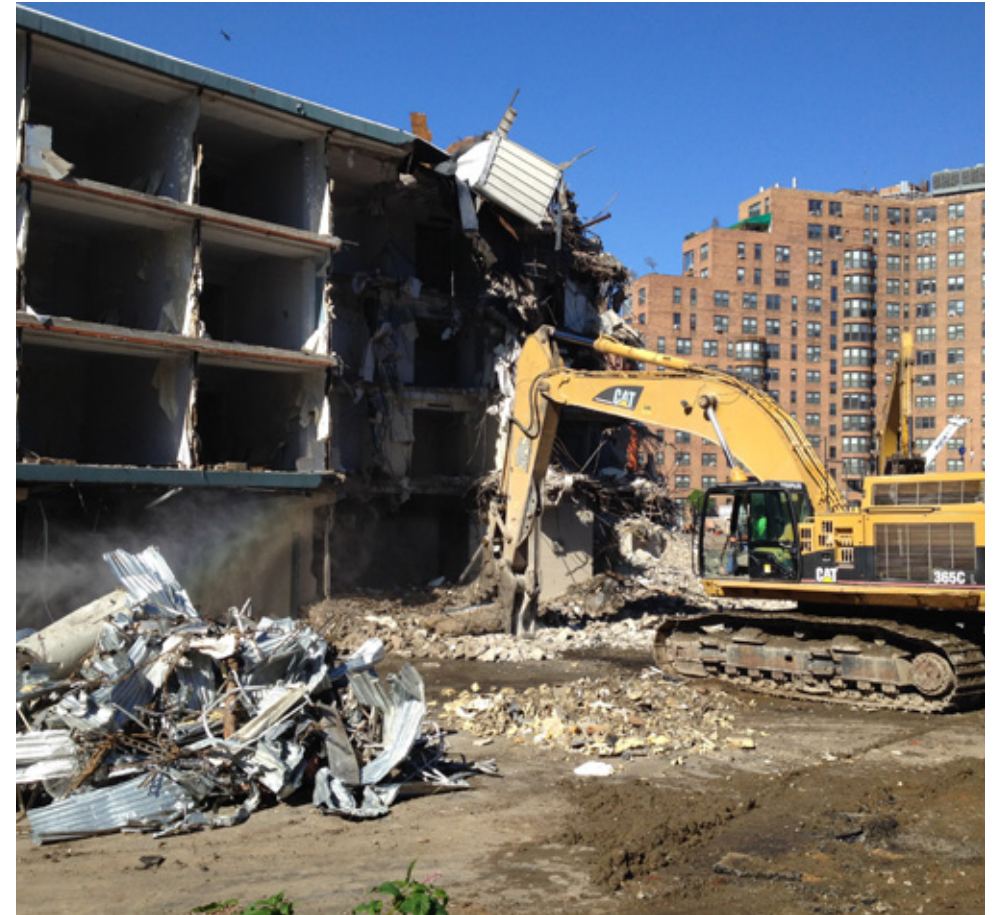
Fig 4.11 Demolition and material sorting. Philadelphia, PA, USA
