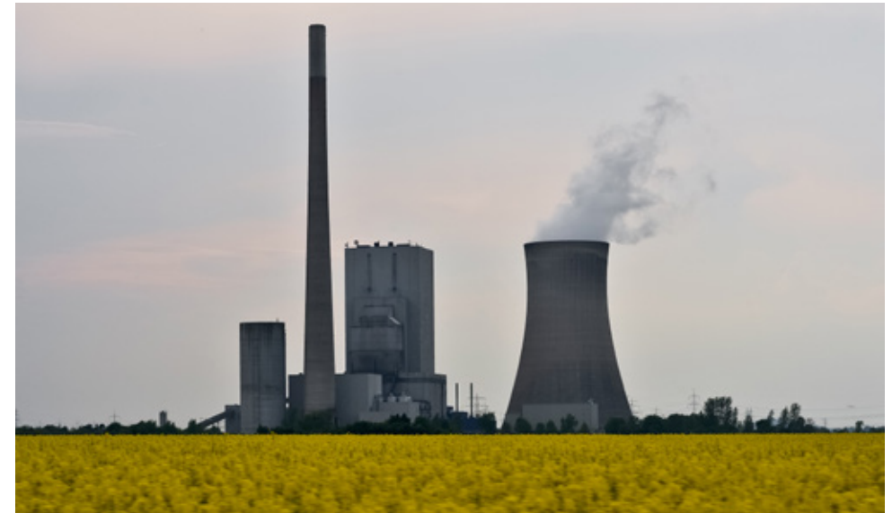
Fig 6.2 Coal fired power station in Mehrum, Germany
